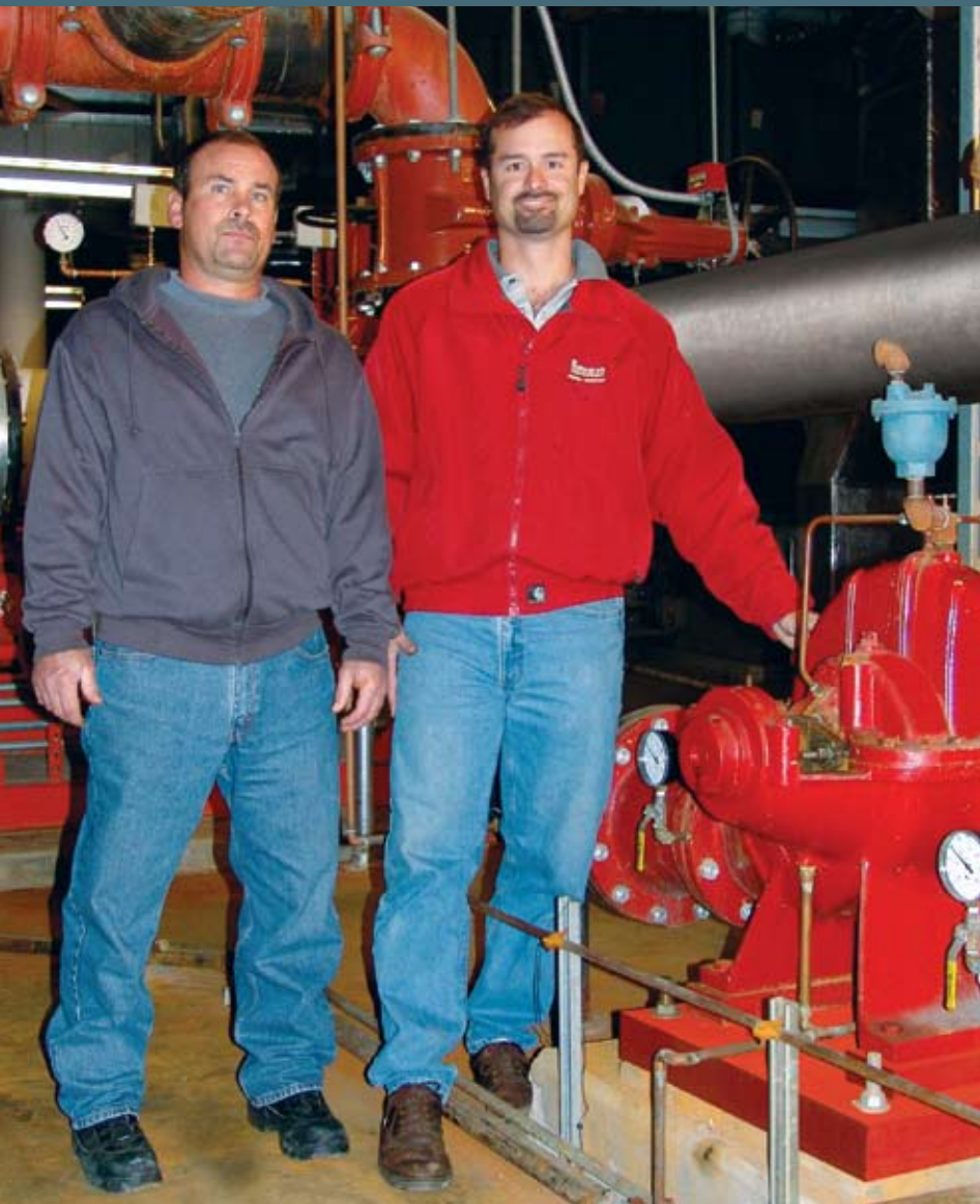
Kevin Waters (left) and Greg Trombold of Trombold Equipment Company.
